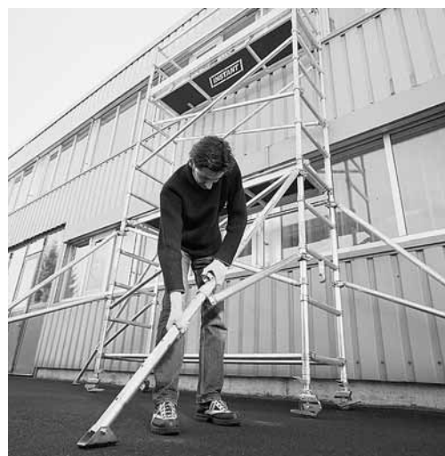
Fig. 3: The assembly instructions specify the height from which supports must be fitted.
