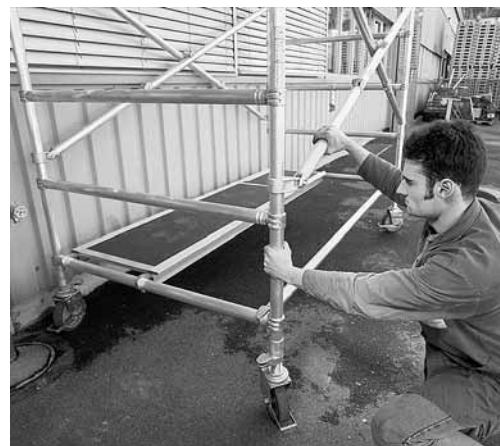
Fig. 1: Fault-free mobile scaffold towers are essential for safe working.
