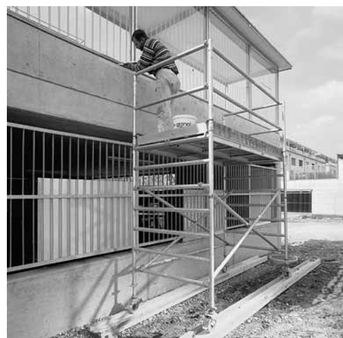
Fig. 2: A firm foundation prevents the castors from sinking in without warning.
