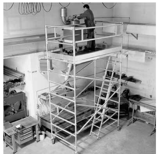
Fig. 6: Missing guardrails and defective boards may cause people to fall from a height.
