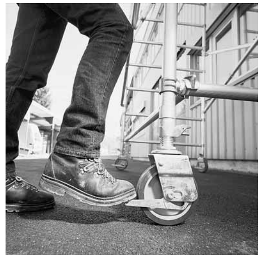
Fig. 4: Castors must be secured to prevent the mobile scaffold tower from accidentally starting to roll.
